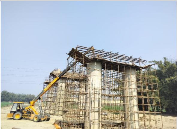
Pier Cap Shuttering
