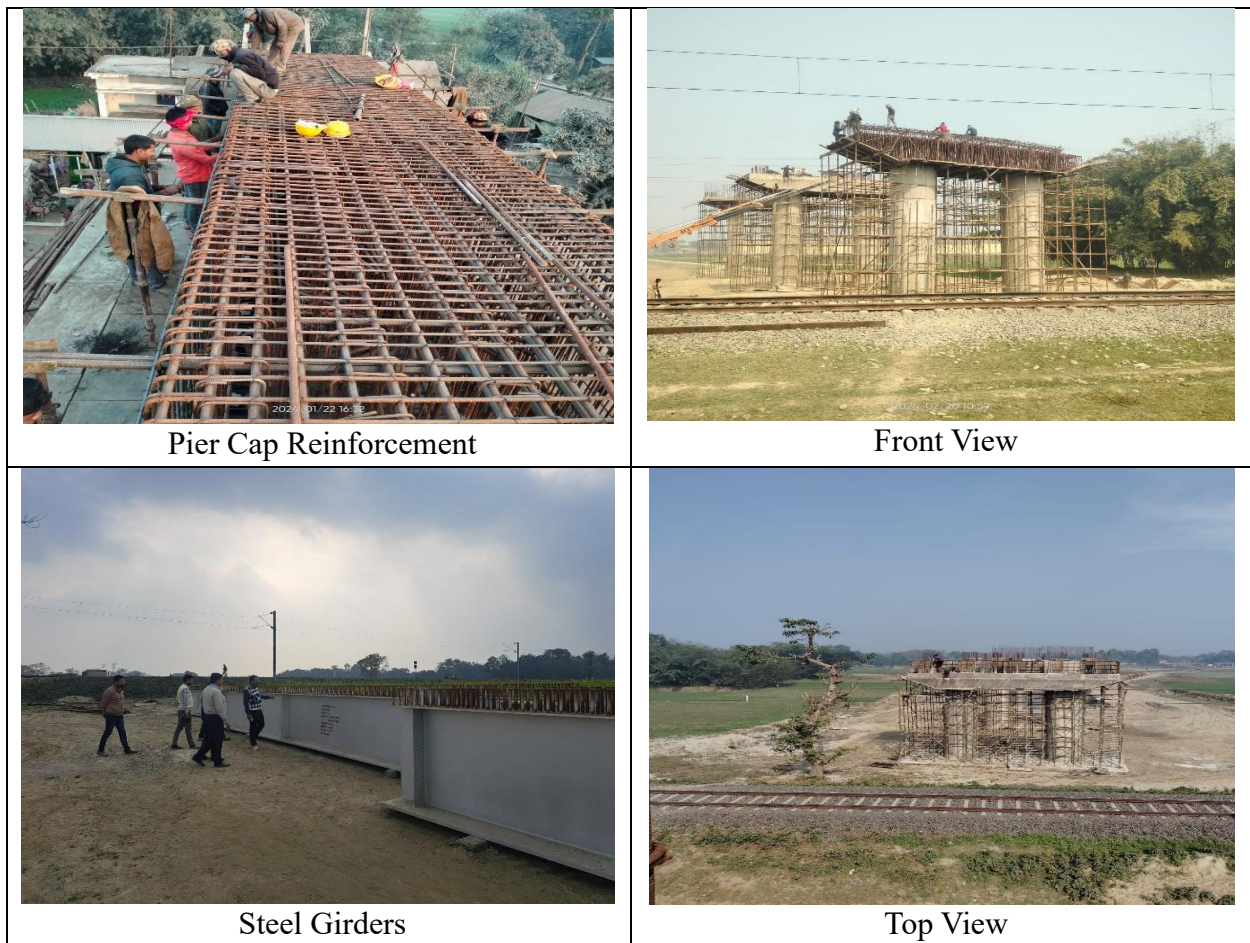
Fig. 2: R.O.B. at Madhepura Bypass on NH 107
