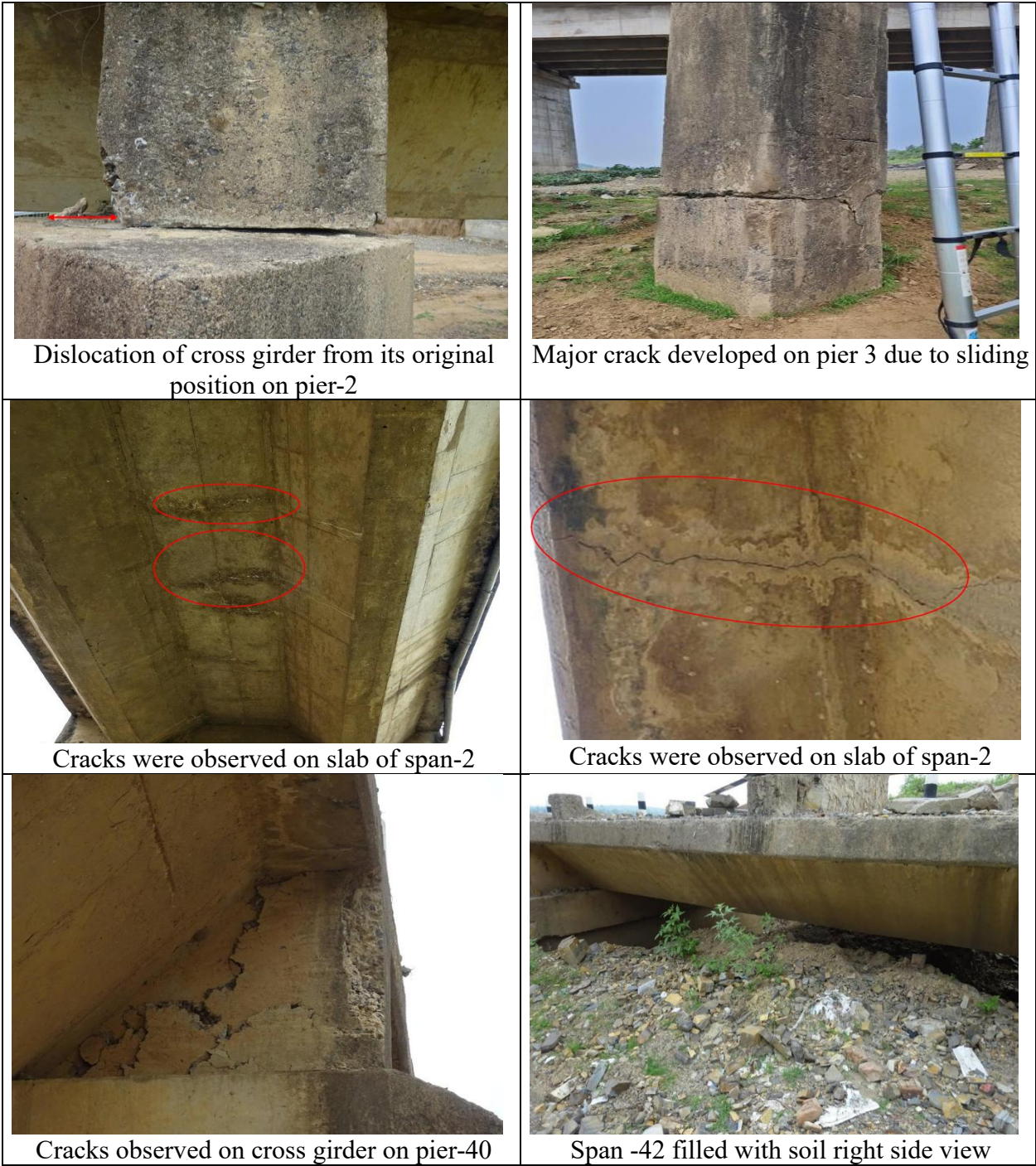
Fig. 3: Sone River Bridge Rewa Madhya Pradesh
